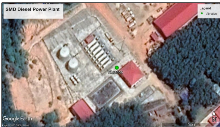
Figure 6- 10 Locations of Vibration Measurement Point
